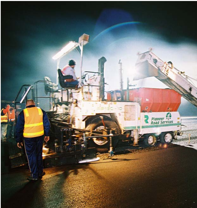
Brisbane Airport main runway overlay, Brisbane
