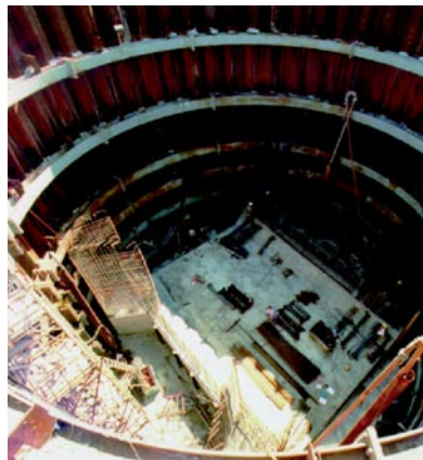
New Southern Railway, Cooks Crossing, Sydney
