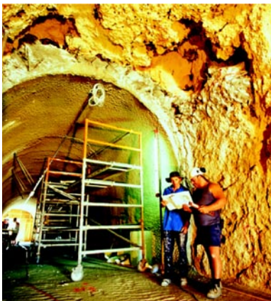
Whalers Tunnel, Perth
